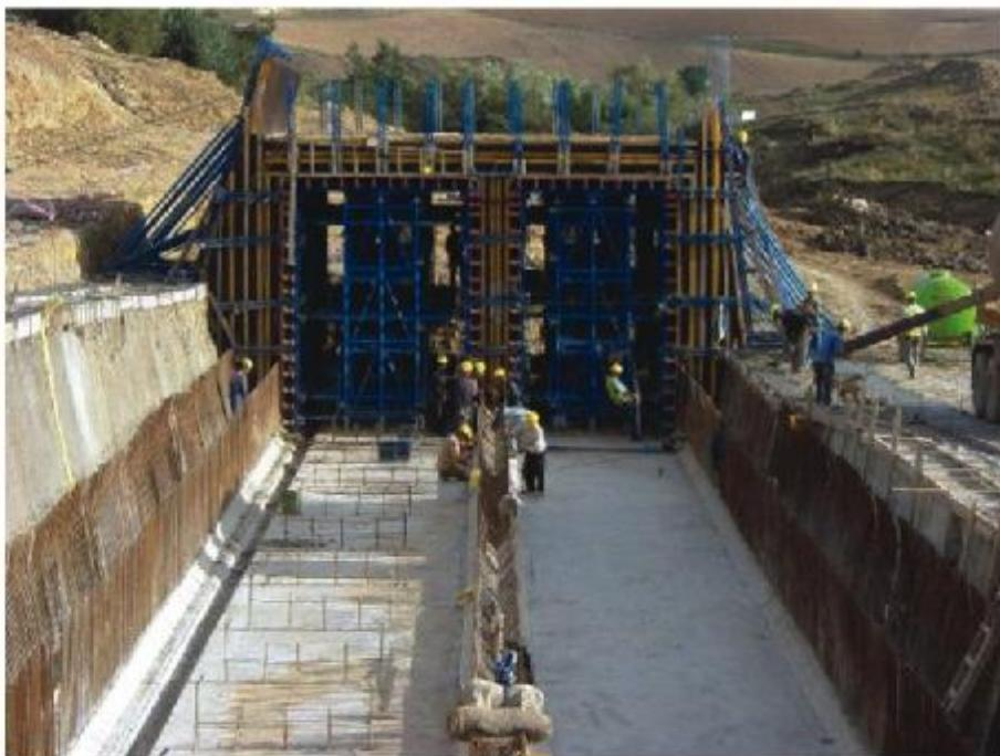
Custom Box-Culvert formwork by using standard formwork elements, highly adjustable, highly flexible and still reusable for other forming purposes.
