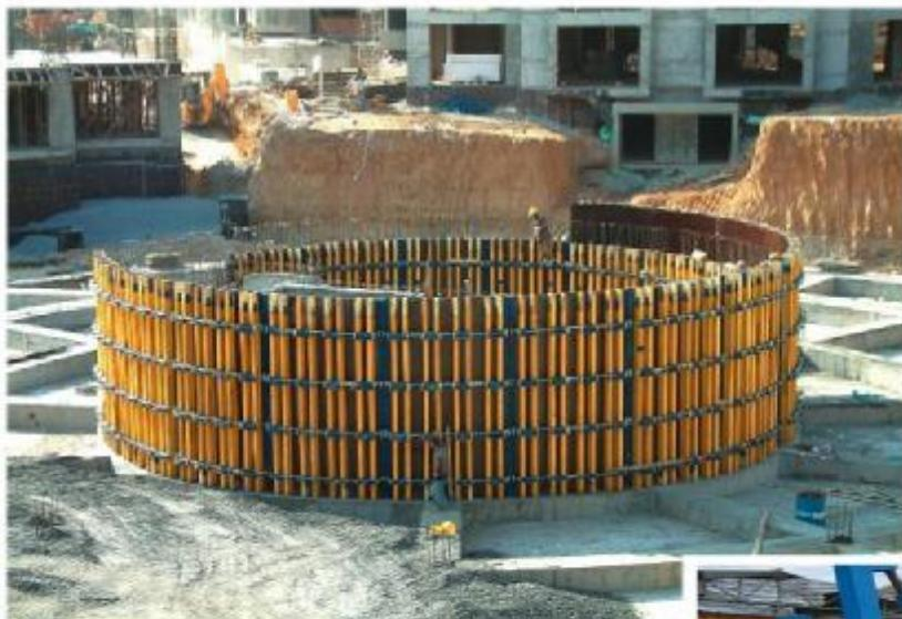
TMS Roundex is a radially adjustable formwork system designed especially for sewage plants, water tanks, car park ramps, silos, pools and even the most complex architectural circular walls.
