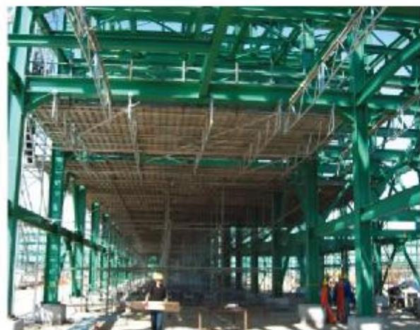
Custom made Pipe-Rack Suspended Scaffolding for GATE.
