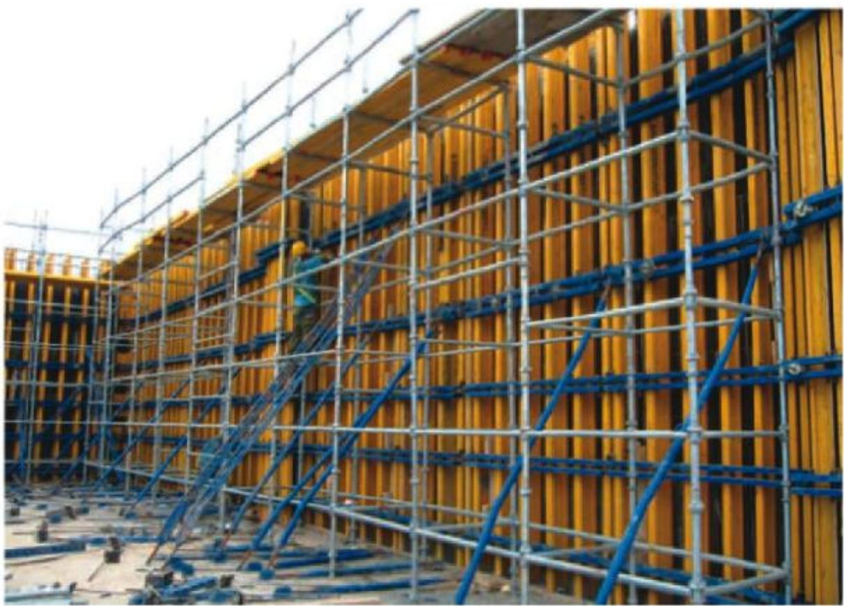
Being used as work scaffold at the back of SIMPEX wall formwork.
