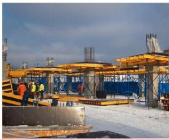
Table around column-heads, for the recessed soffit height.
