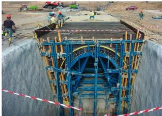
Injection Tunnel Formwork
