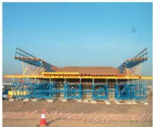
MK-H 150 Shoring System together with Multix adjustable waling System.
