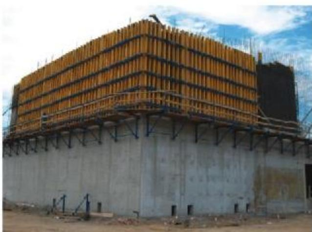
SIMPEX Wall Formwork with TRK 160 Climbing Systems
