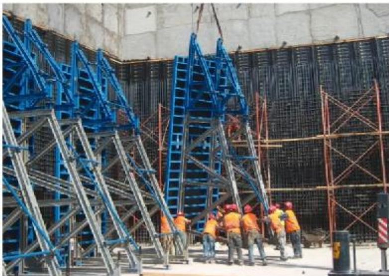
A technological warehouse project in Istanbul. VİNCİ 80 Wall and Column Formwork at 11.20m height. Multix RAM single sided braces and TRK 250 D climbing brackets are used against existing insulation walls.
