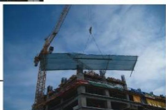
Standard safety Platforms could be ganged and crane handled
