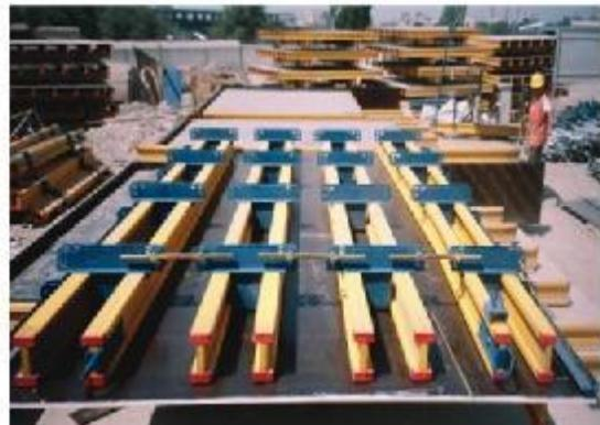
Roundex panels are assembled with plywood, HT 20 timber beams, special walers and the push-pull type spindles between them.
