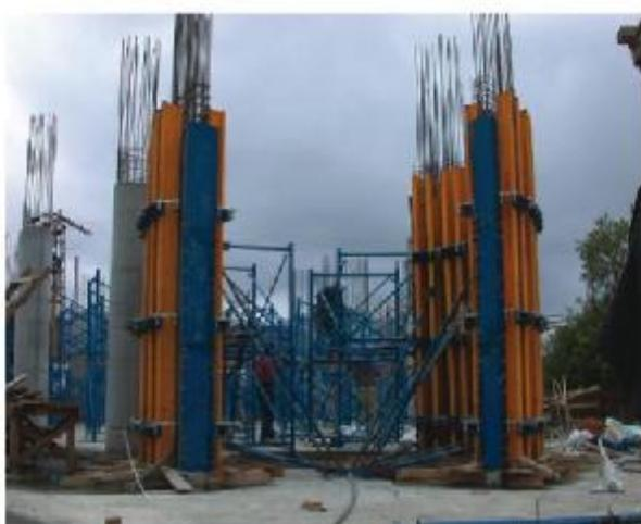
TMS ROUNDEX, an adjustable formwork system for radii larger than 1.2 m forming circular structures, especially the ones with varying radii have always been costly, if not difficult from the contractors view point.
