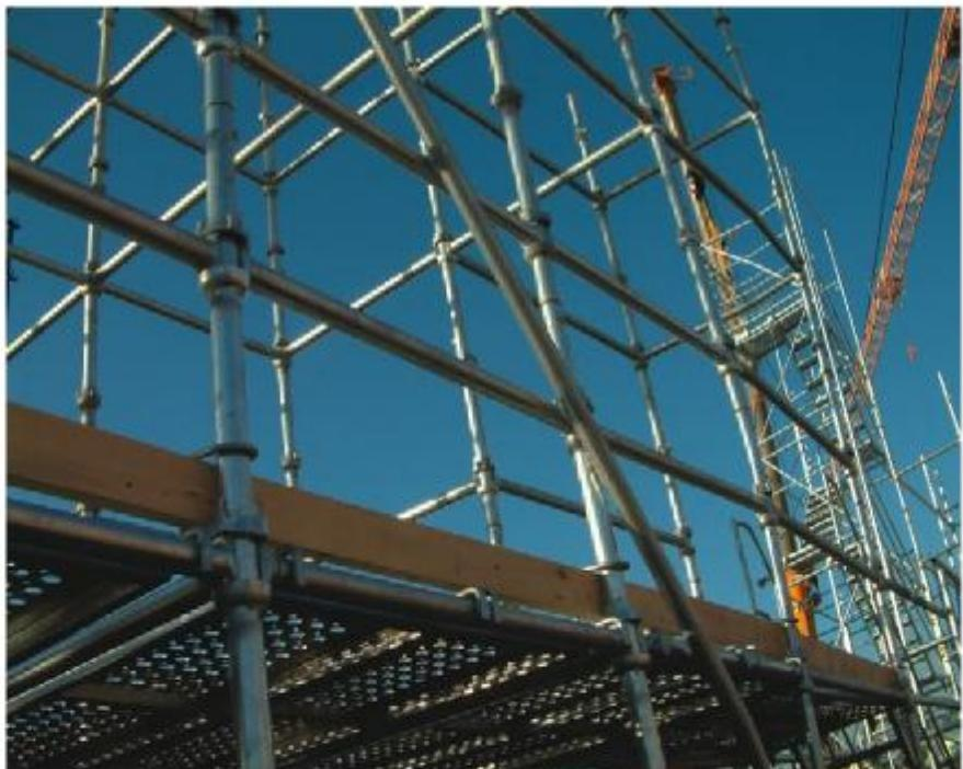
Tri-fold safety with toe-guards and two level handrails.
