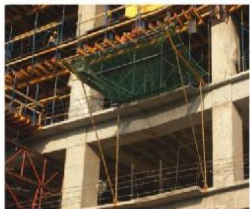
While nets with larger diameter ropes and larger meshes serve for fall-protection, another layer with thin but tight meshes could stop falling tools, debris etc.
