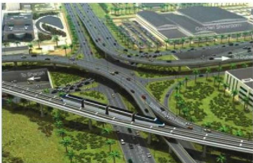
Two new junctions over Al Khail Road has been constructed for easing up the heavy traffic load. Each junction consists of two 200m long bridges and 600m long ramps for heavy trucks.
