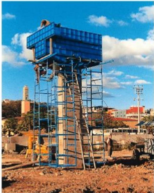
Socket foundation formwork for precast column application
