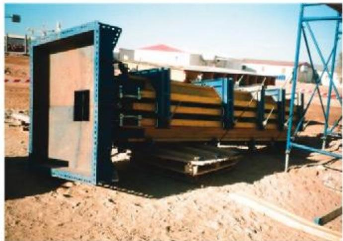
Battery form for precast concrete piles.
