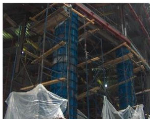
Circular Column Formwork around structural steel columns of a high-rise building at Moscow City, for fire-proofing the critical columns.
