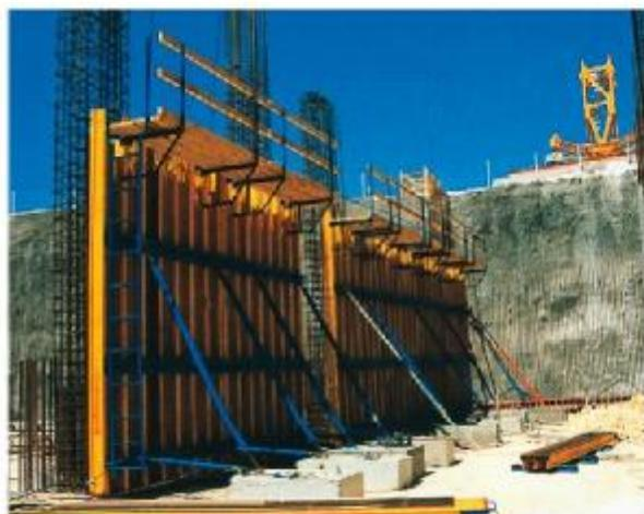
Istanbul Olympic Stadium retaining walls & mega-structure walls at civil works, SIMPEX Wall Formwork.
