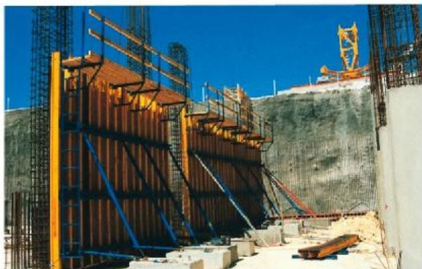
Concrete weight blocks for anchoring the push-pull props.
