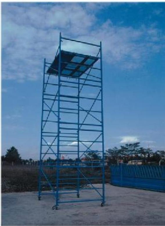
According to BS 5973 the height of a mobile platform cannot exceed 3 times the minimum base width at open air, in closed areas the maximum height could be 3.5 times the min. Width of the base.
