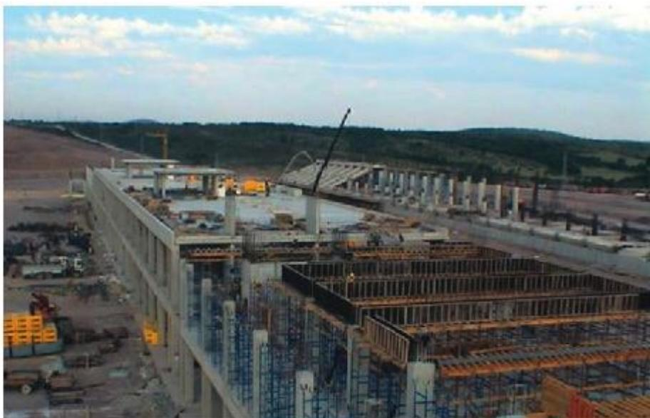
With the load bearing capacity - i.e. 49,6 kN/leg at h=5,5m - of the system, bracings between the towers are minimal, allowing for significant distances between the towers even under thick slabs.
