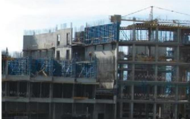
VINC'I 80 Wall Formwork and Slabflex Slab System as been used in this 70.000 sqm project.
