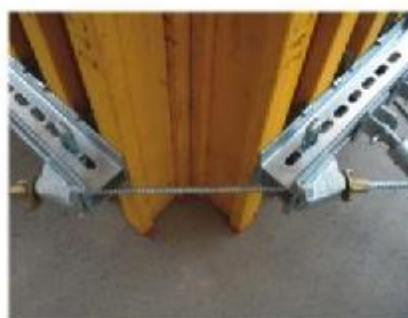
Corner-shoe detail for angular corner tensioning
