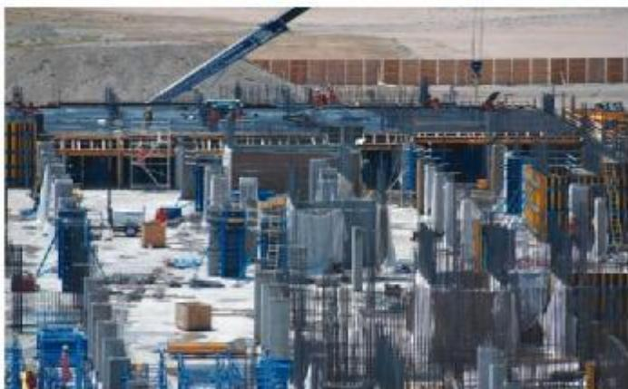
Depending on the height and type of building , a combination of MK-H 150 Table Form Slabflex and Flexdeck Systems are applied for the slabs.
